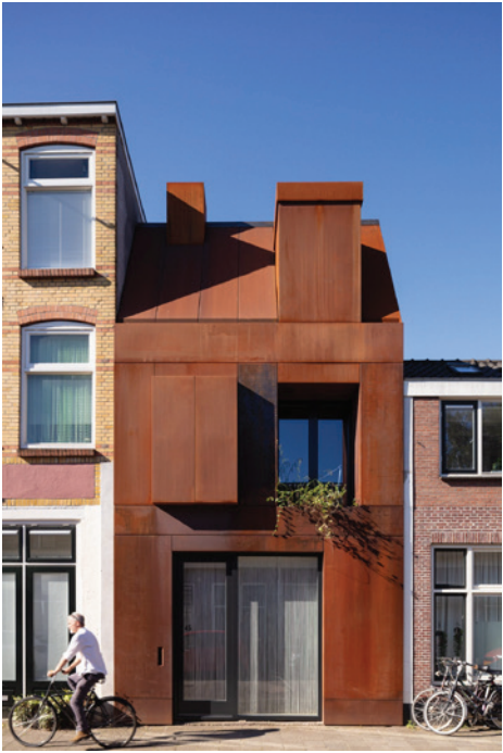
Zecc Architecten - garage infill conversion, Utrecht
